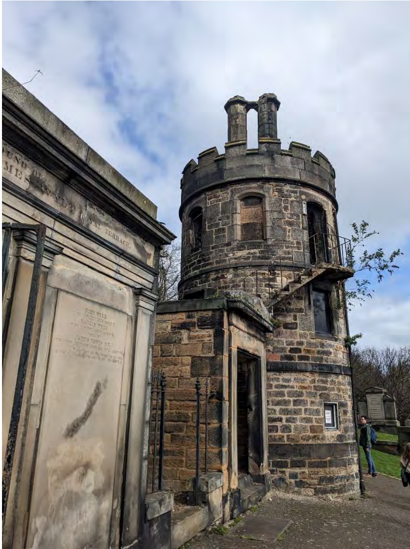
Watch Tower from west
