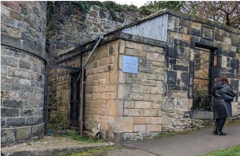
Adjacent outhouse from southeast
